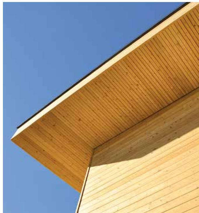
Larch is weatherproof and can be installed outdoors in its natural form. Over time, the cladding or terrace turns silver. Larch is highly valued by those who prefer a long-lasting solution. The big bonus with this is the limited need for maintenance.
