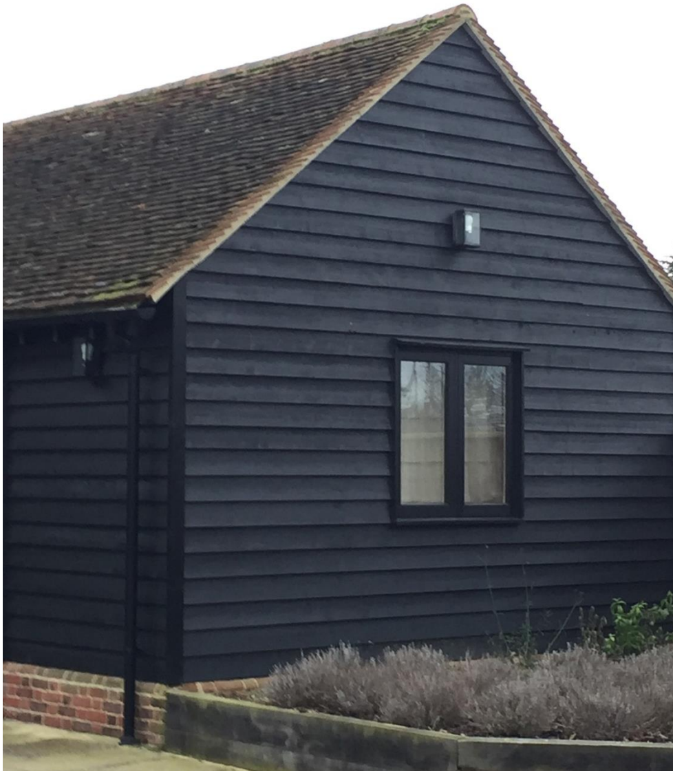
Figure 1. Painted planed timber exterior cladding in use
